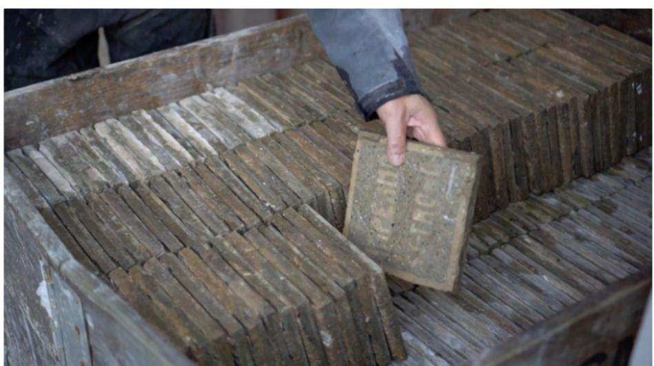
**EN** - We mechanically cut away the mortar residue on the underside of the tile to make it easier to reinstall.
