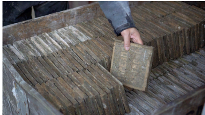
Cleaning mortar residues and sorting quality
